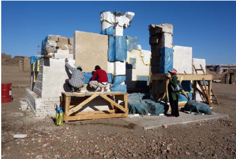
Fig. 45: Coarse spray plaster on the front side of Osiris Nesmeti Temple (photo: © A. Krekeler).
