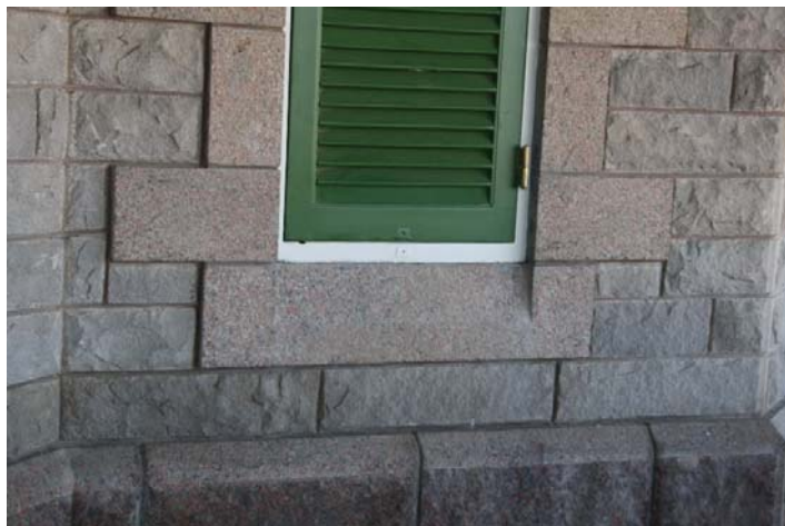
Fig. 1a, 1b and 1c: Aswan Museum Elephantine, granite blocks of the west elevation, varnish stains before (top), during (middle) and after cleaning (photos: M. Fahmy © DAI Cairo).
