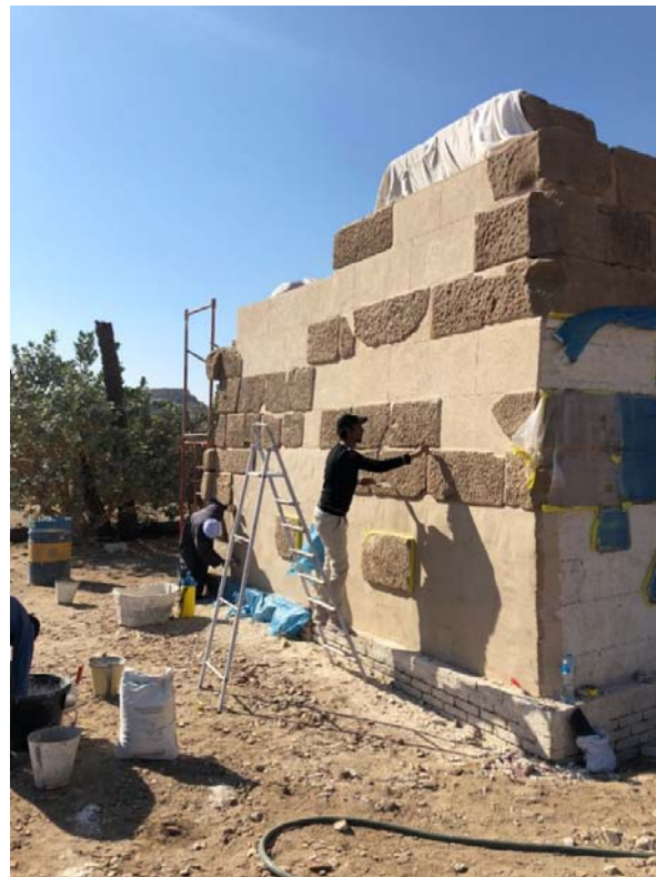
Fig. 46: Levelling plaster and finishing plaster with incised joints on the backside of the temple (photo: © A. Krekeler)
